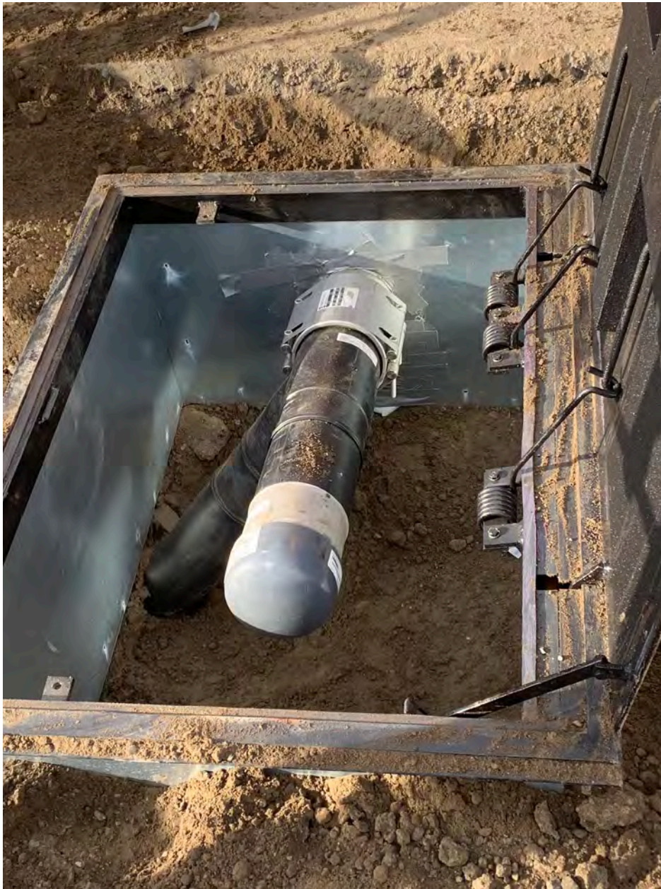
Photograph 9: View of HSVE-01 well vault installation and stub-out, looking west.
