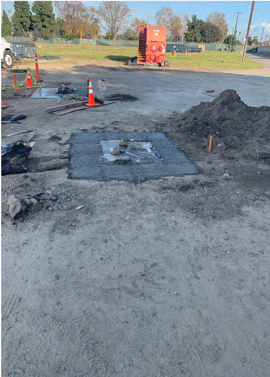
Photograph 10: View of HSVE-01 (front) and BS-03 (back) vault completions, looking east.
