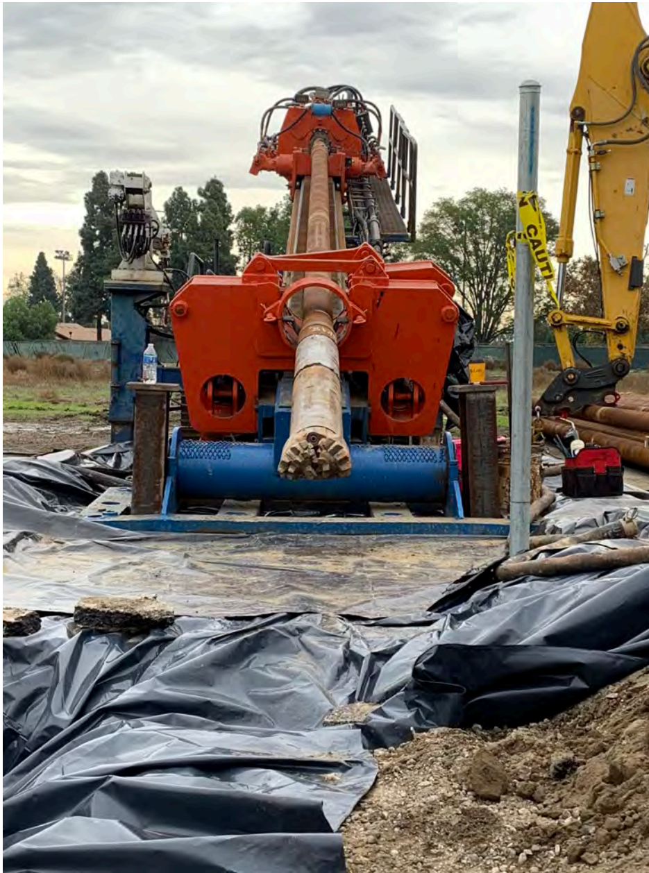
Photograph 1: View of drill rig (American Augers DD210), looking east.
