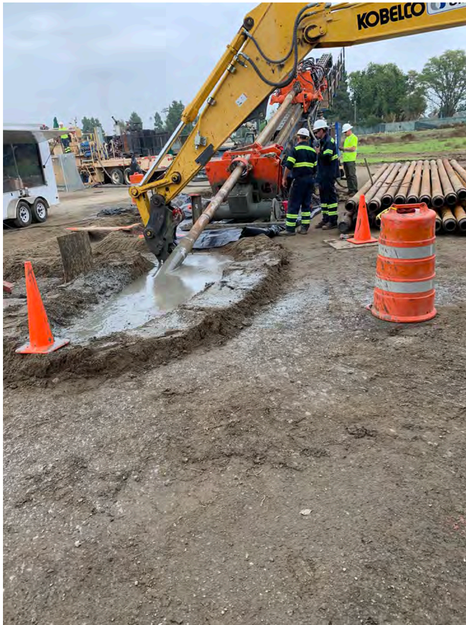
Photograph 7: View of HSVE-01 boring progression, looking east/northeast.
