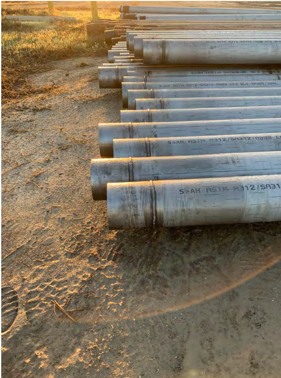
Photograph 5: View of 6-inch-diameter blank and slotted stainless-steel casing for HSVE-01, looking north.
